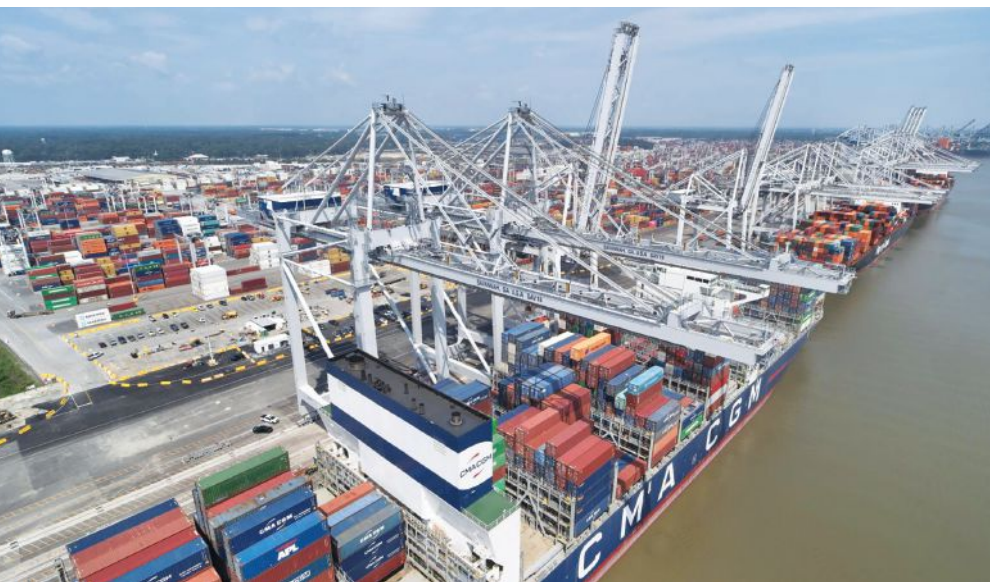
Increased Capacity: Garden City Terminal's container Berth 1 was recently renovated
